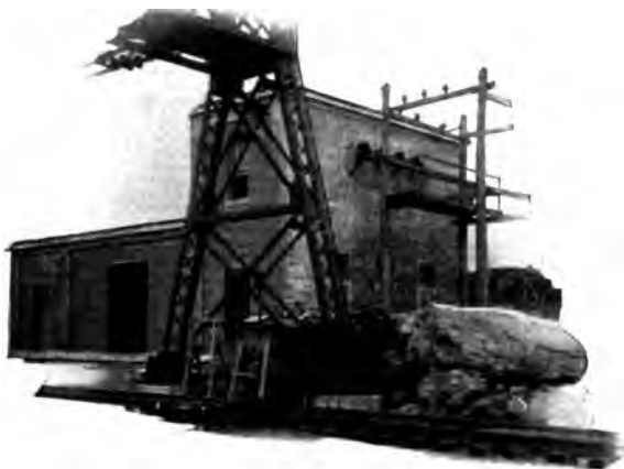
Signal Sub-Station of the New York, Westchester & Boston
